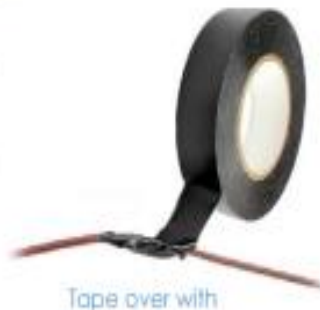
Tape over with insulating tape
